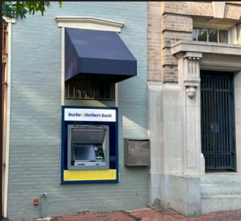
This ATM is inappropriate because it is located on a highly visible location on King Street.
